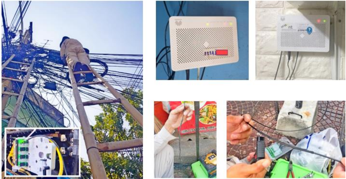
Figure 37. Long insulation connection point in Samranrat area
