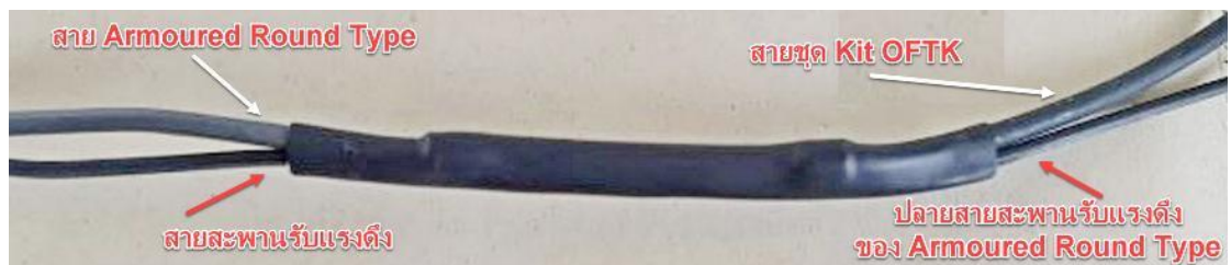
Figure 25. Wrapping the bridge cable with a tensile force-receiving tube at the fiber optic connection points.
